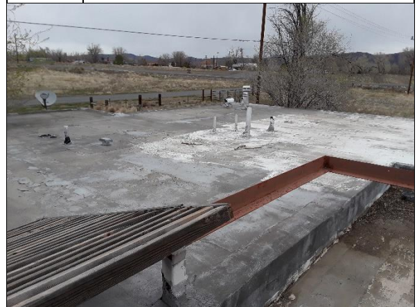
5. ACM Roof View Looking West
