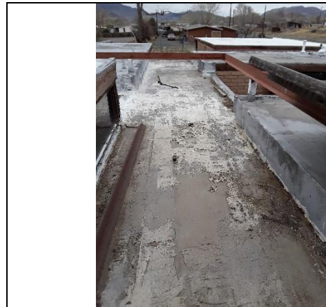
4. ACM Roof View Looking North
