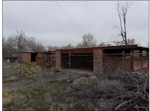
11. General View of Garage
