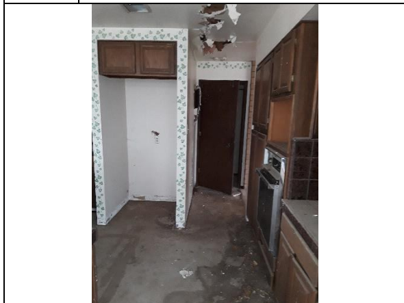
3. RACM Sheet Flooring Remnants In Kitchen
