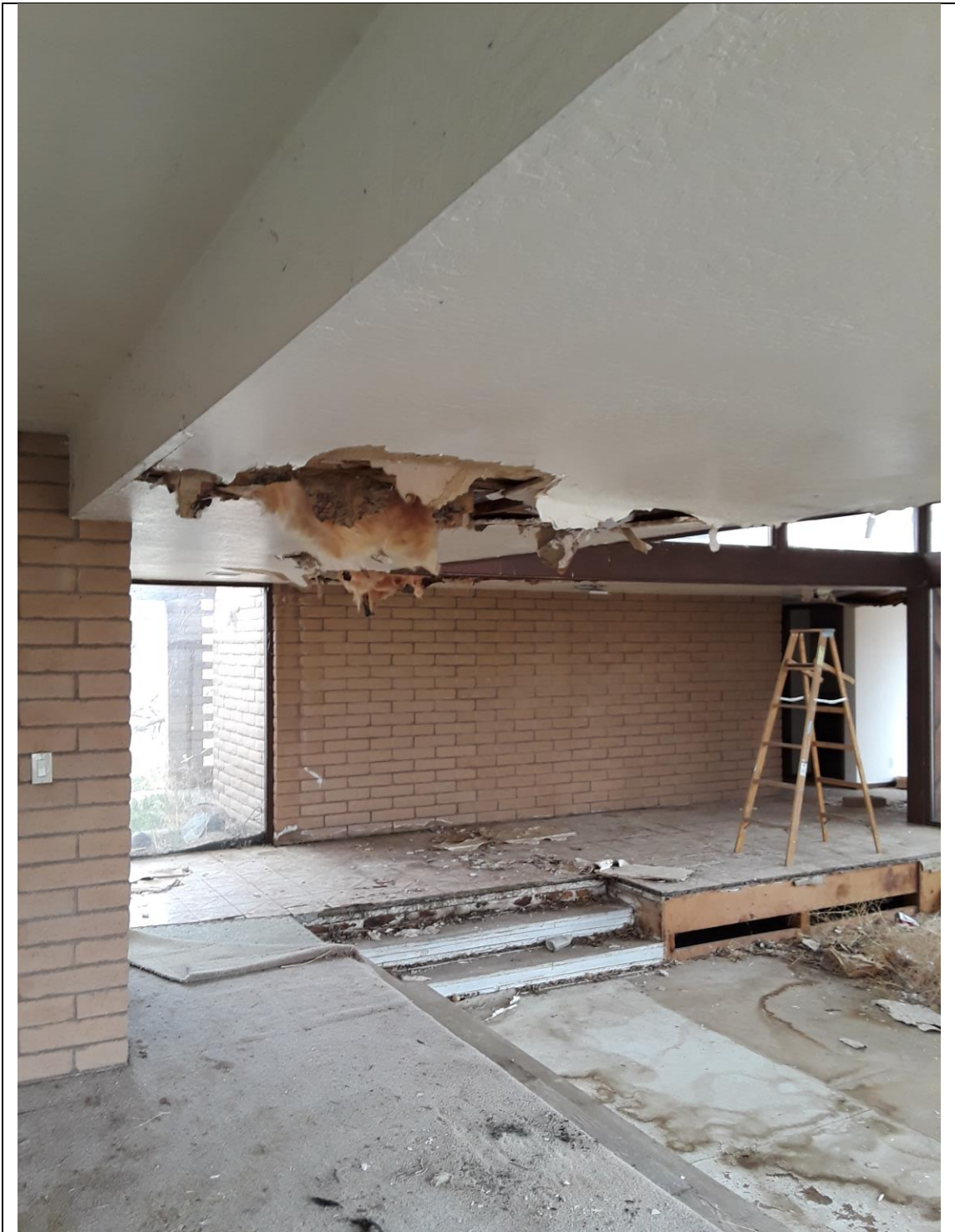
Photograph #2: Lead containing beige floor tile (glaze) in main hallway.
