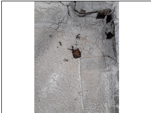
1. ACM Roofing Material With Silver Paint
