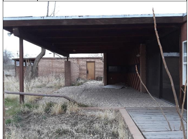
12. General View of Side Patio and Behind Garage
