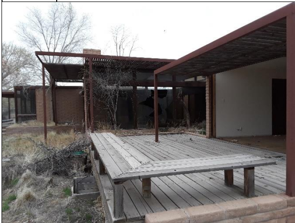
9. General View of Back Patio Deck
