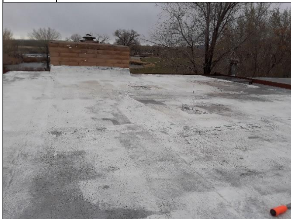
2. ACM Roof View Looking East
