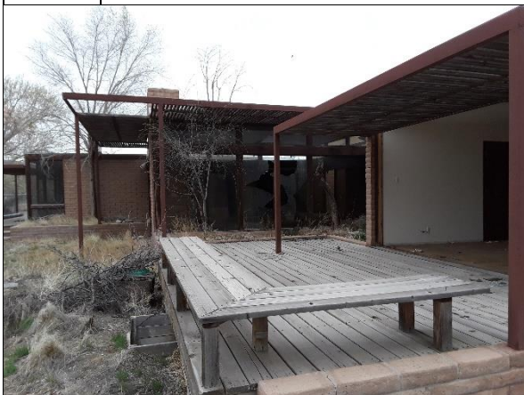
9. General View of Back Patio Deck
